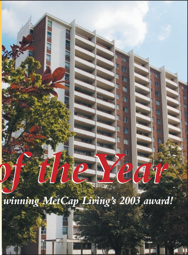
15 Tangreen Court – Part of the Yonge Village Apartments
